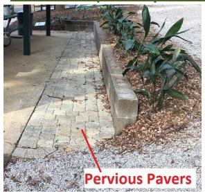
The pavers around the pavilion are pervious and designed much like a sponge with millions of tiny pores that allow water to soak through them and into the ground below. This provides a nice firm surface much like a traditional patio but reduces the amount of stormwater runoff.
