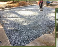
Excess water in the narrow paver strip drains through a pipe to a Dry Well under the BBQ pad. The main patio drains through the gravel beneath then through the 3 pipes in the wall to the rain garden.
