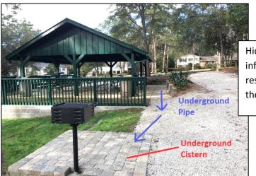
Hidden beneath the new BBQ pad lays a Dry Well (a.k.a. infiltration chamber or cistern). A dry well is basically a large reservoir where stormwater is stored until it has time to soak into the ground and help recharge our drinking water aquifer.
